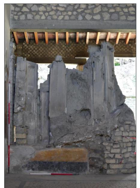
Fig. 6: Plaster cast (OPL\_007) of two shuttered, bivalve windows (left and centre), and the left bifold of a quadrivalve door (right) in the southeast corner of *oecus* (15), the famous 'peacock room'.
